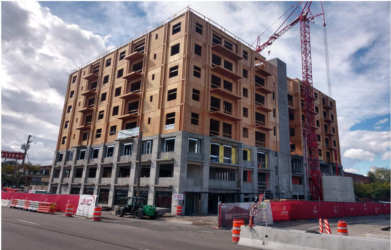
Figure 2. Structures like this 5-over-3 podium building near Salt Lake City, Utah, can use wood harvested from the WUI to provide dwelling units in increasingly densified urban corridors while helping to reduce standing tree densities in nearby forests. This FRTW could also be used in structures built in the WUI, too.
